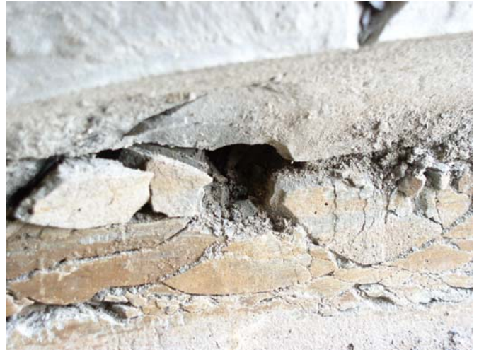
Figure 8 – Entry hole to Cement and Shale
